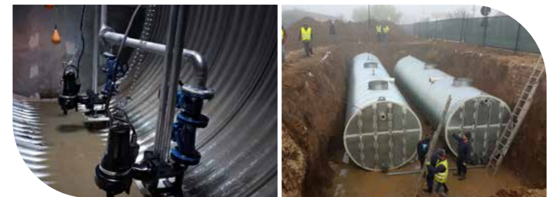
more than 1,000 m 3 capacity / stormwater retention in corrugated steel tubes / fast installation / sustainable solutions
